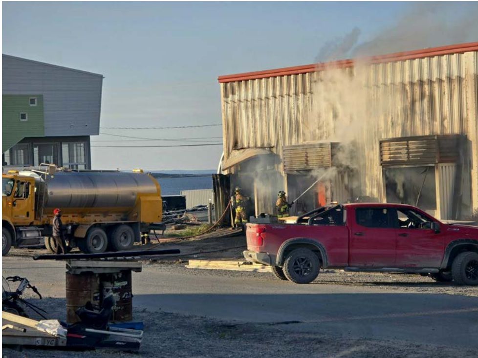
Smoke rises from the Naulait Men’s Association building in Umiujaq after it was destroyed by fire in the early morning of Sept. 2. (Photo courtesy of Qalingu Napartuk)
